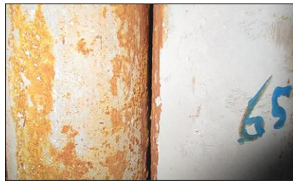
Figure 4. Tangent tube of a D-style boiler division wall.
