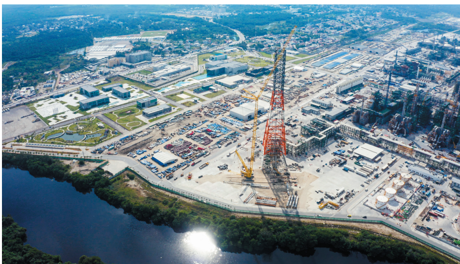
Figure 4. Case study 3 – demountable flare system during derrick construction.
