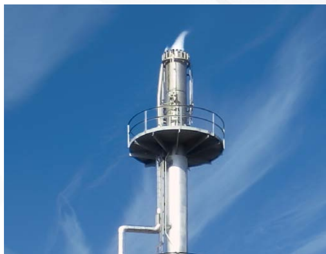
Improper application of steam
