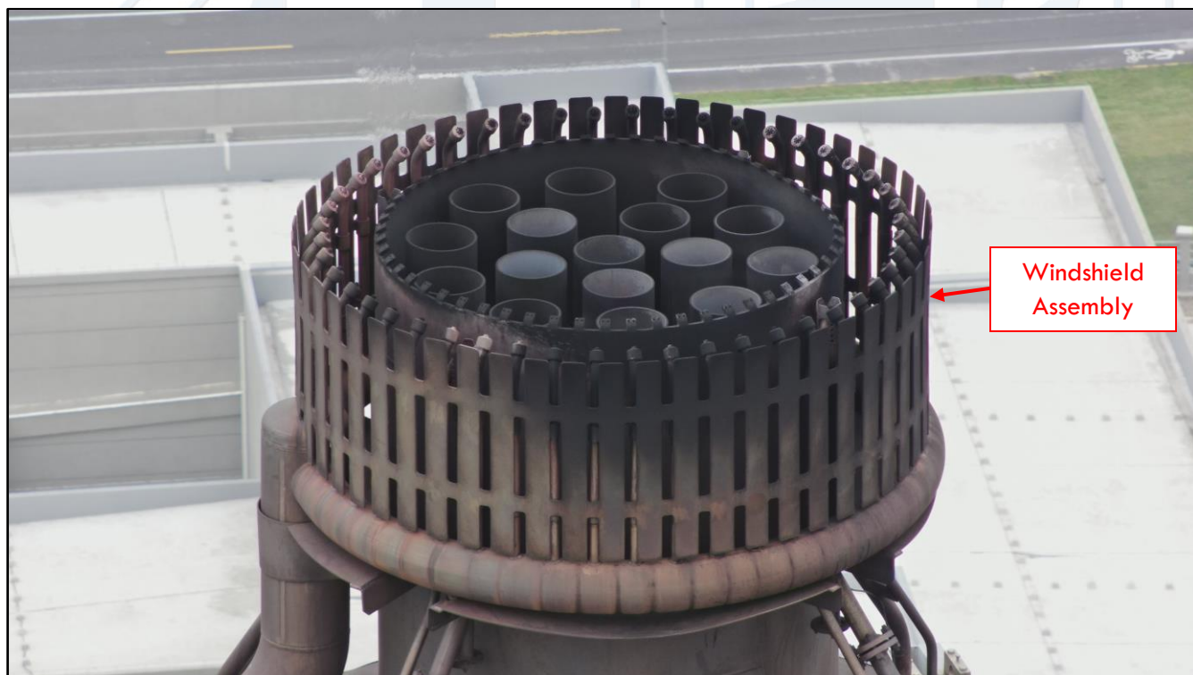
FIGURE 03 – Perimeter steam injection appears to be in fair condition. No deformation is detected on the upper flare tip barrel. Soot deposits are observed on the windshield assembly.
