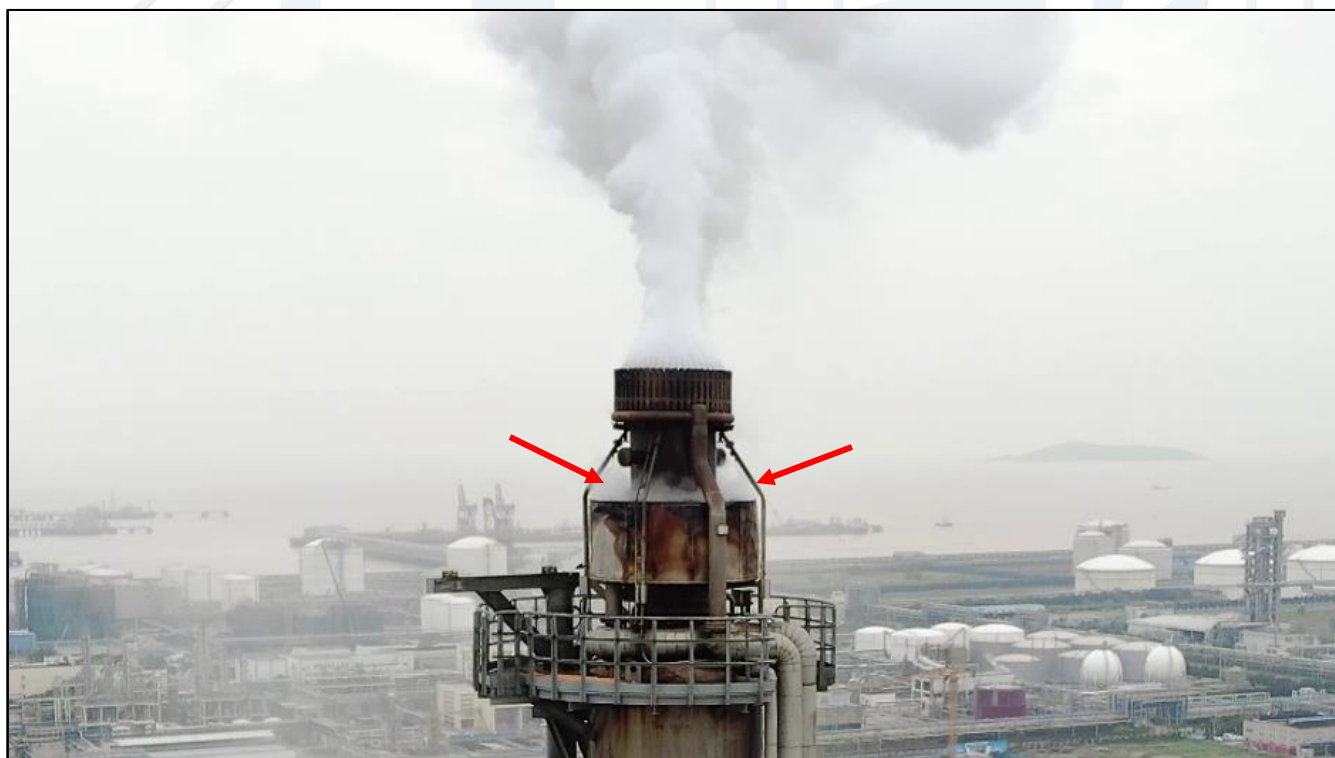
FIGURE 11 – Steam condensation exiting the noise muffler; this indicates breakage in steam tubes. Smokeless capacity has been compromised, and there is the potential for tubes to break apart and fall into the molecular seal assembly.
