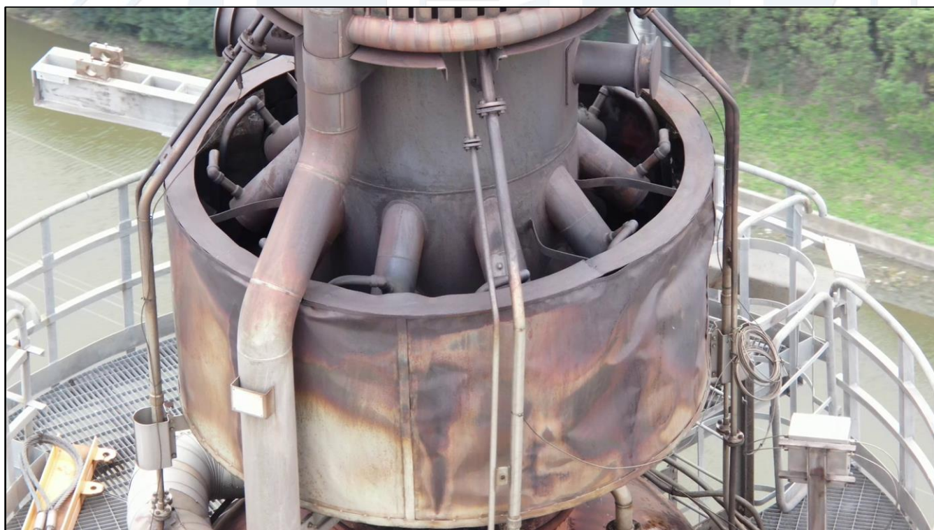
FIGURE 09 – Thermocouples are directly exposed in the heat affected zone. Zeeco recommends running thermocouples in tubing or conduit to prevent failure.
