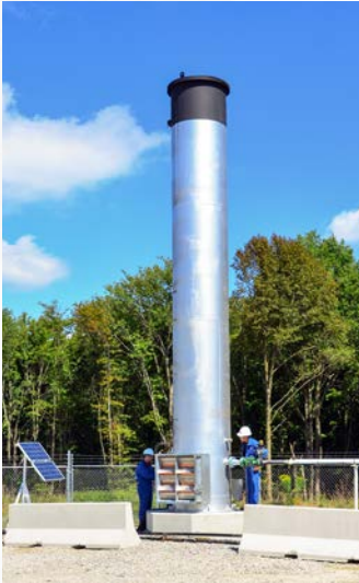
Operated as Flare, Incinerator, or VCU
