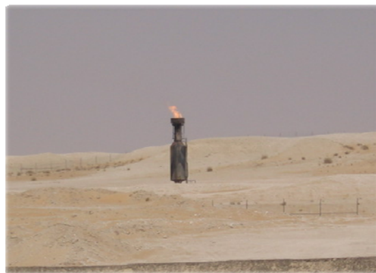
Figure 11. Jobsite C With HPAAS Upgrade
