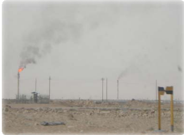
Figure 8. Typical Smoking Flares in Saudi Arabia
