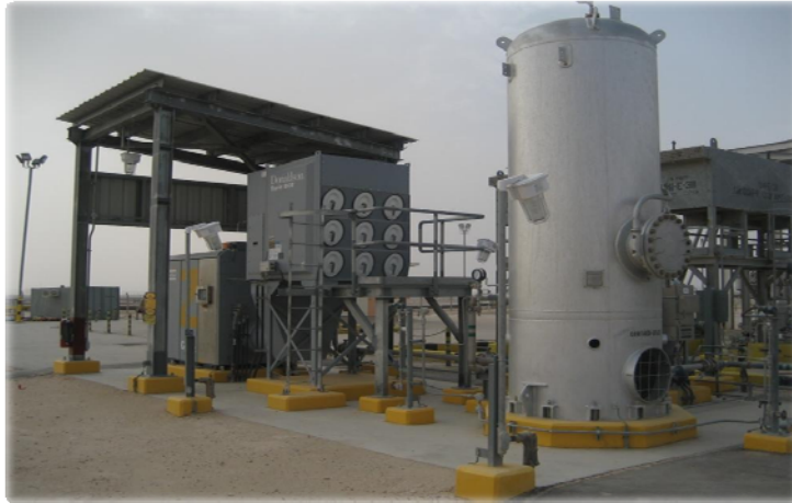
Figure 7. Smokeless Air System for Typical HPAAS Installation
