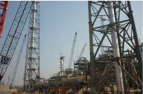
Erection of a sulfur tail gas thermal oxidizer vent stack. Zeeco’s field support engineers are fully equipped to assist in all of your equipment erection and commissioning efforts.
