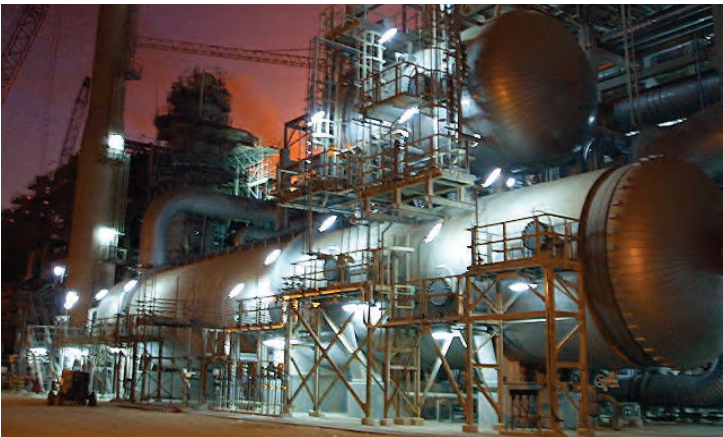
SRU Tail Gas Thermal Oxidizer with firetube waste heat boiler and steam drum. One of nine similar systems supplied by Zeeco.
