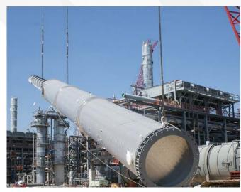
Incinerator Stack Single-Point Lift
