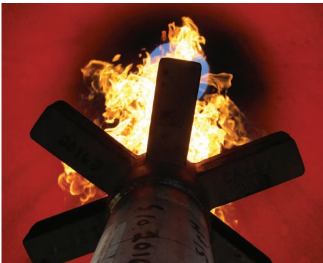
Internal view of a ZEECO enclosed combustor
